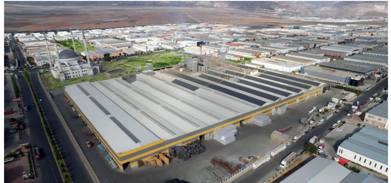
RAVABER Kayseri Manufacturing Plant, Turkey
